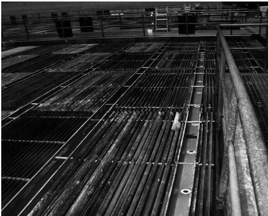
Fig. 9 : Condenser tubes in the power plant circuit after one year of continuous treatment. No visible scaling has occurred.
